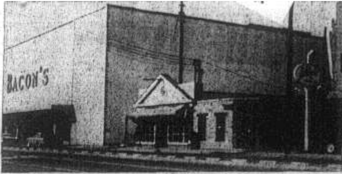
A familiar scene to most people in St. Matthews but it has changed as the photo at right will show. The two buildings right of Bacon's have come down to make way for the firm's expansion. Barbara Clarke, a woman's apparel store, Bechtel Interiors, and a restaurant occupied the buildings until recently.
